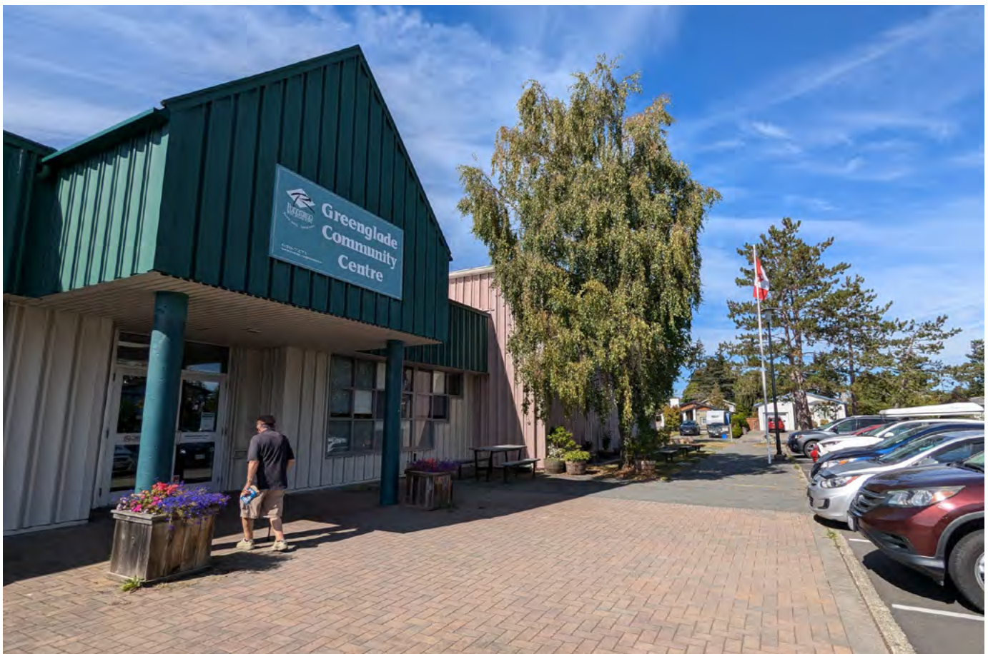
Greenglade Community Centre front entry
